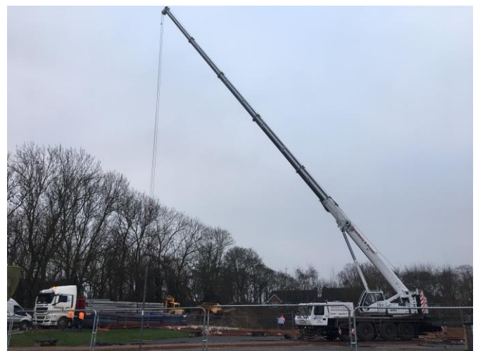
Foundations for the new building
